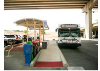
The VIA Metropolitan Transit University Park & Ride Center
